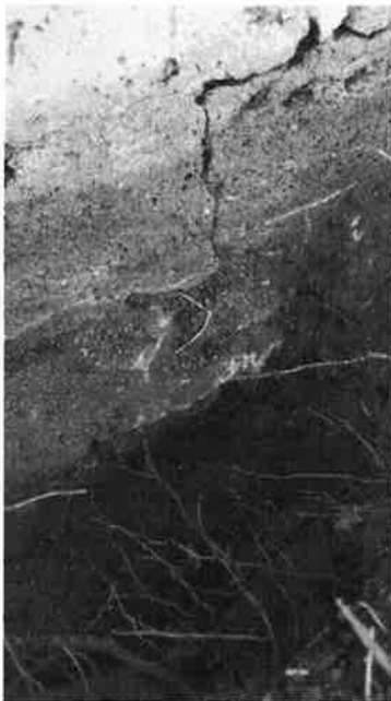
Excavation at crack behind tree 5
