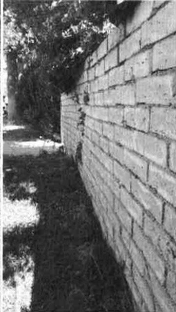
Wall not plum/straight along Webster Near Tree 4
