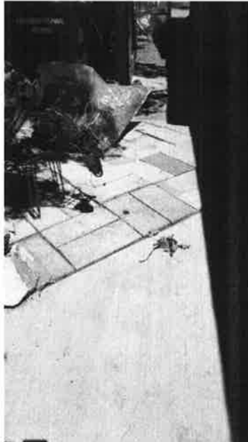
Pavers in patio/walkway
