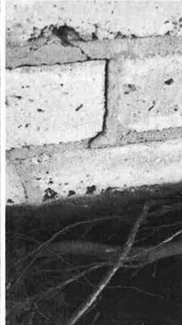
Excavation at crack behind tree 5
