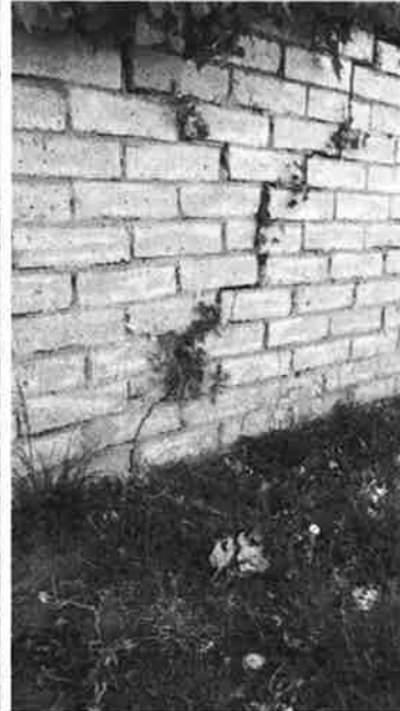
Wall not plum/straight along Webster Near Tree 4
