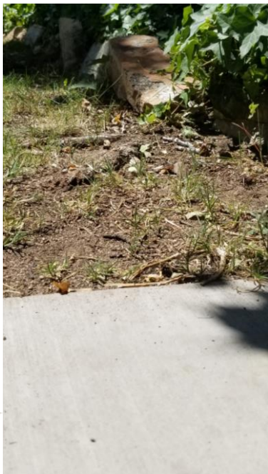
Surface root inside yard
