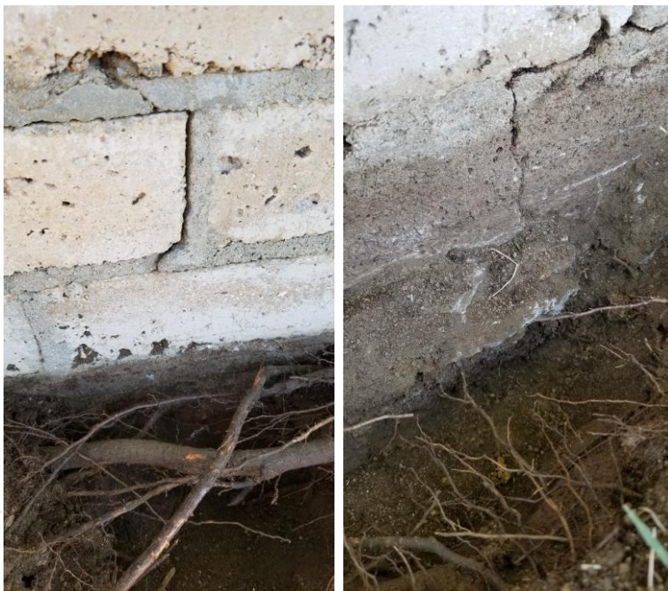
Hand excavation near Tree 5
