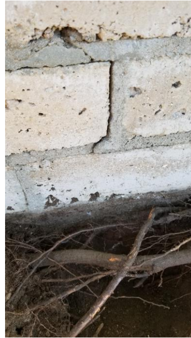
Excavation at crack behind tree 5
