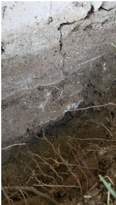
Excavation at crack behind tree 5
