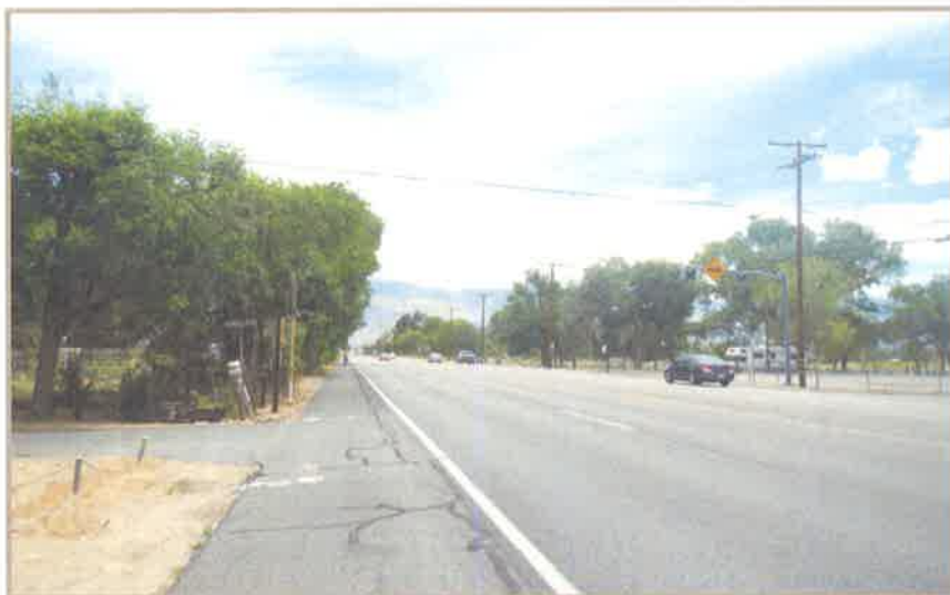
Lack of pedestrian facilities
