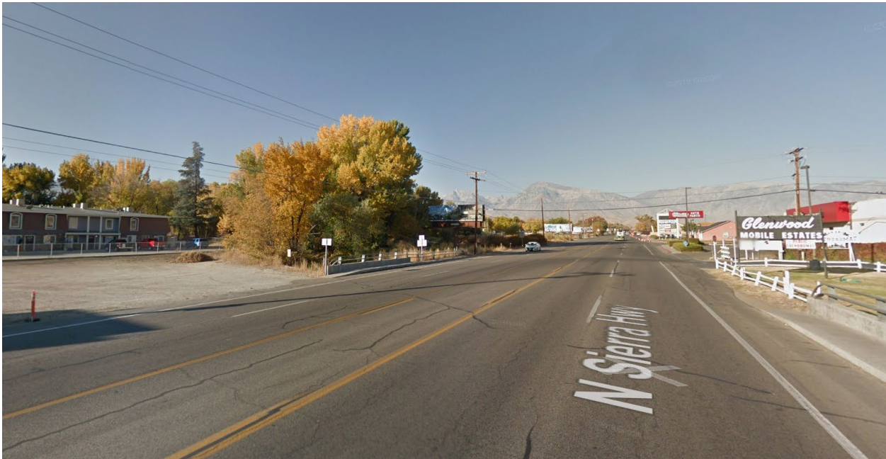
Figure 4 - Sidewalk gaps on north (right) and southbound sides of U.S. 395 at Bishop Creek Bridge.
