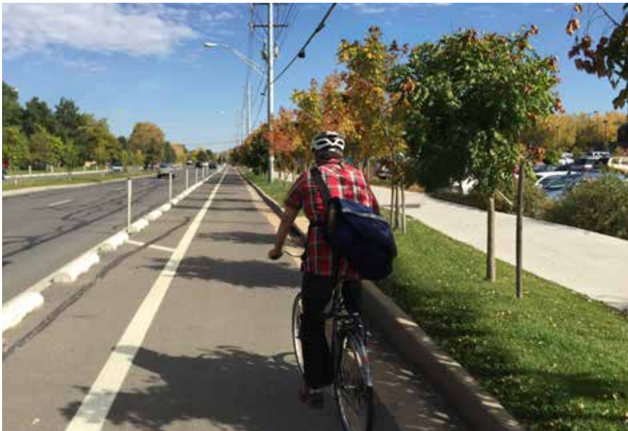
An example of a Class IV separated bike lane in Boulder, CO. In this case the bike lane is separated from the roadway by striping, parking blocks, and flexible vertical delineators.
