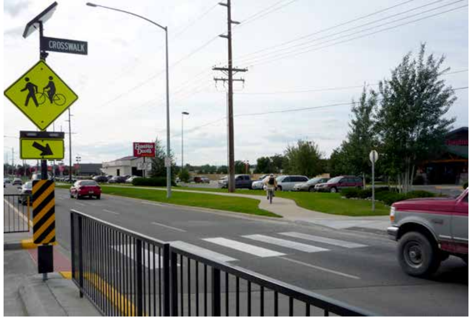
An example of a high-visibility crosswalk with a rectangular rapid flashing beacon (RRFB) in Billings, MT. Source: Nacto.org
