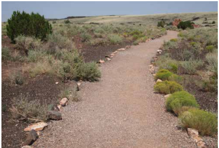
An example of a crusher fines trail lined with native rock in Lomaki Wupatki National Monument, AZ. Source: Americantrails.org
