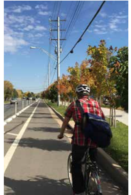
A Class IV separated bike lane using curb stops and flexible delineators.
