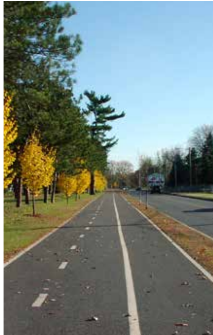
A shared use path striped for separated uses by bikes and pedestrians
