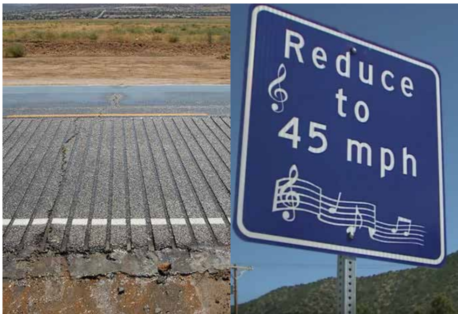
The City of Lancaster, CA is a local example of a musical road. Albuquerque, NM has also installed one along Route 66, pictured above, which plays "America the Beautiful."
