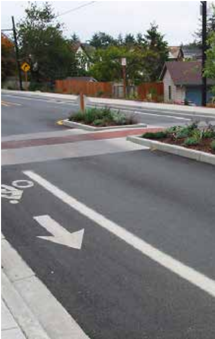
A Class II bike lane near a raised crosswalk with median refuge island
