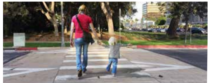
A raised crosswalk slows traffic and allows pedestrians to cross the road safely
