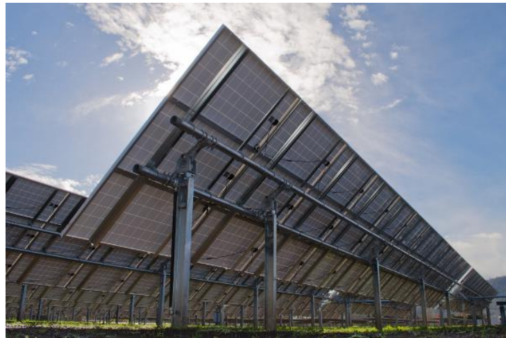
Typical Solar PV Mounting Structure
