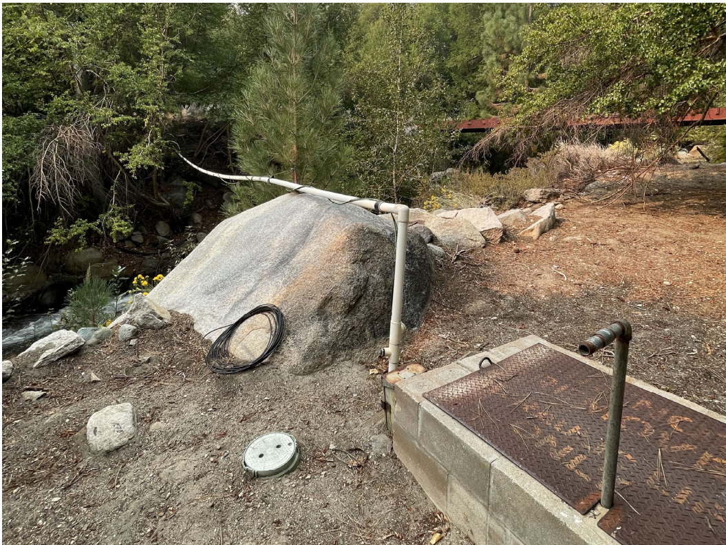
Water supply line crossing over Big Pine Creek
