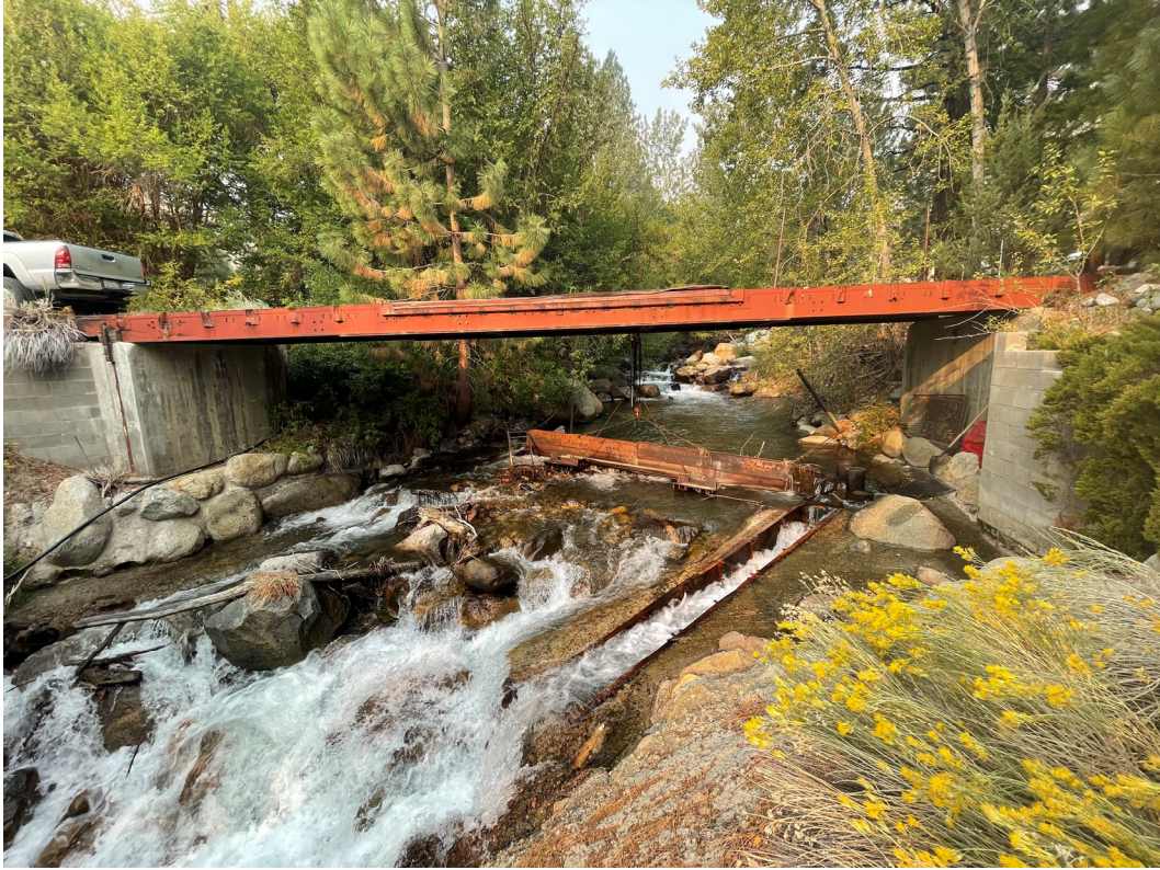
Big Pine Creek looking upstream at Weston access bridge , and water diversion infrastructure.
