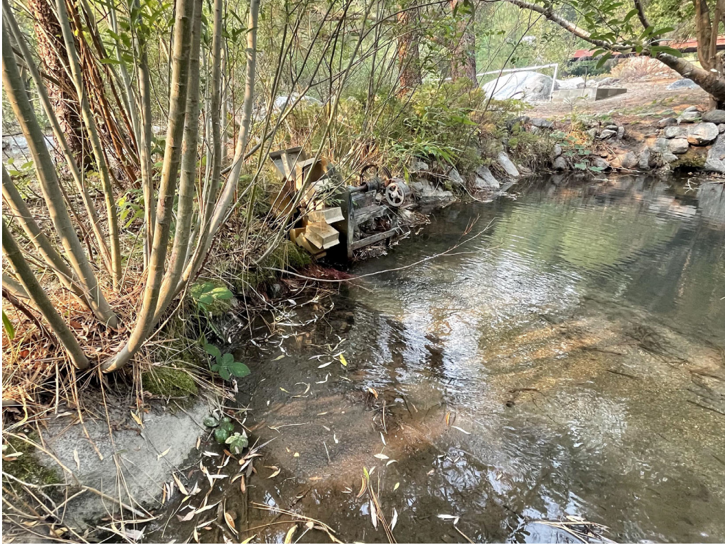
Water supply pond from eastern side looking approximately west.
