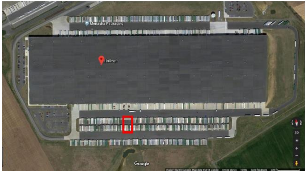
Figure 9.7 Unilver Distribution Center and Trailer Parking Area (Newville, PA)
