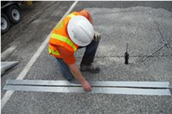
Figure 9.8 Installing In-Pavement Traffic Counter
