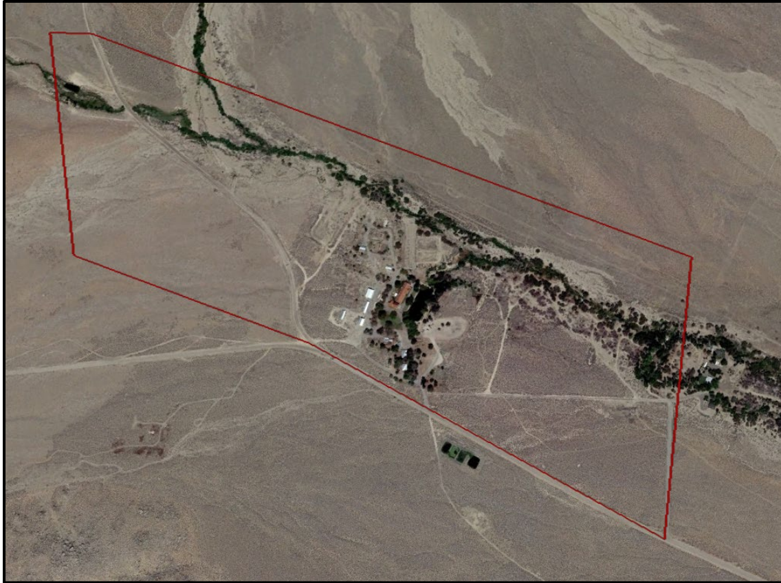
1 2 Figure D.6. There are limited roadways in and out of the community, and all are relatively 3 narrow. The red boundary is the community boundary.
