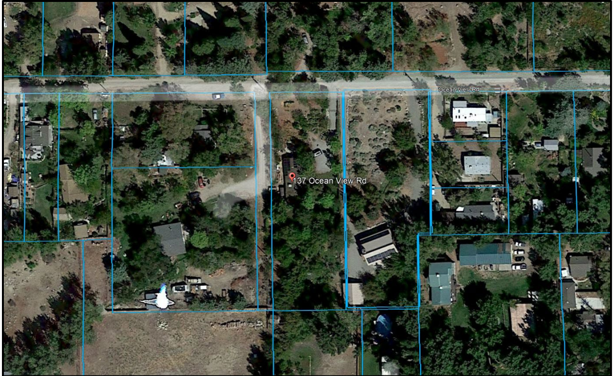
Figure D.12. 137 Ocean View Rd property. Defensible space is fair, although some branches are in contact with the roof and siding. A water tank on the property is accessible via the driveway on the west side. The property is accessible only via Ocean View Rd. The blue boundary is the parcel boundary.
