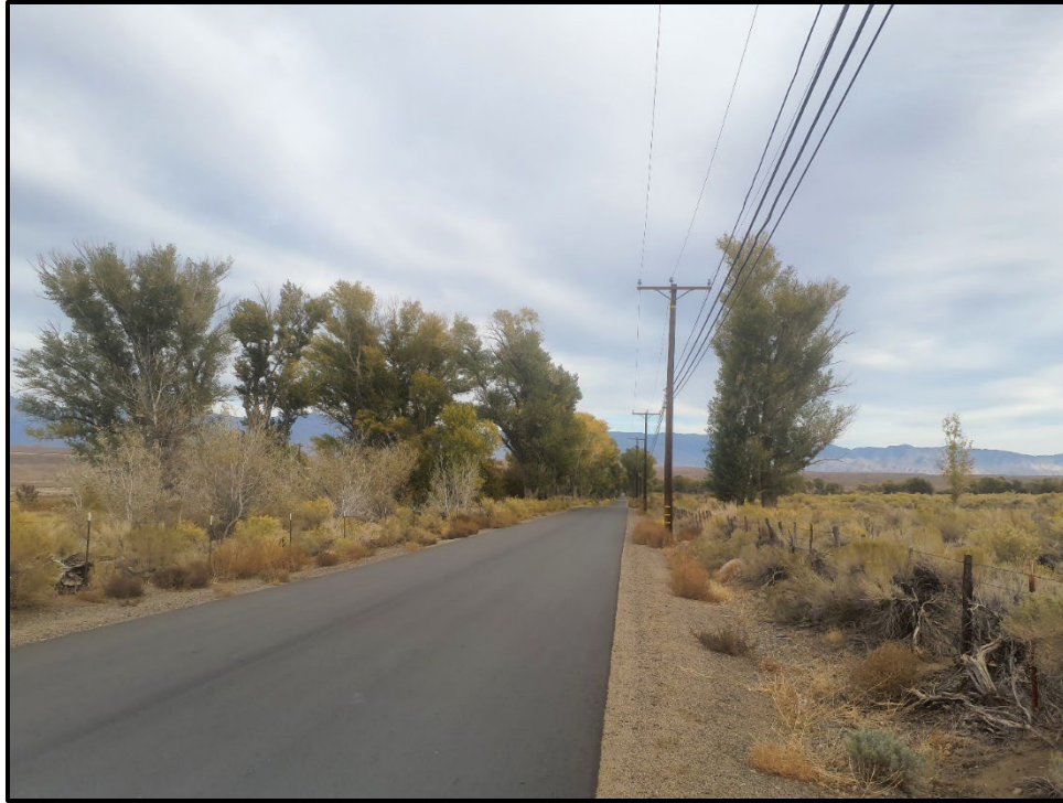
Figure B.3. Birchim Lane; view facing east.
