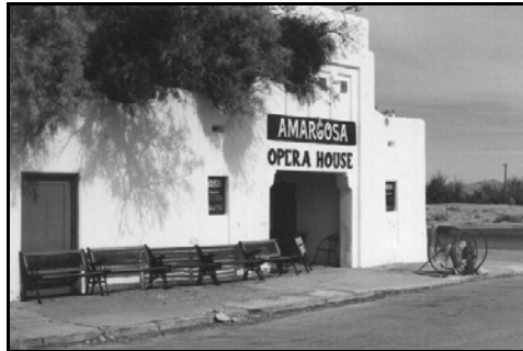
The historic Amargosa Opera House is located in the center of the community.
