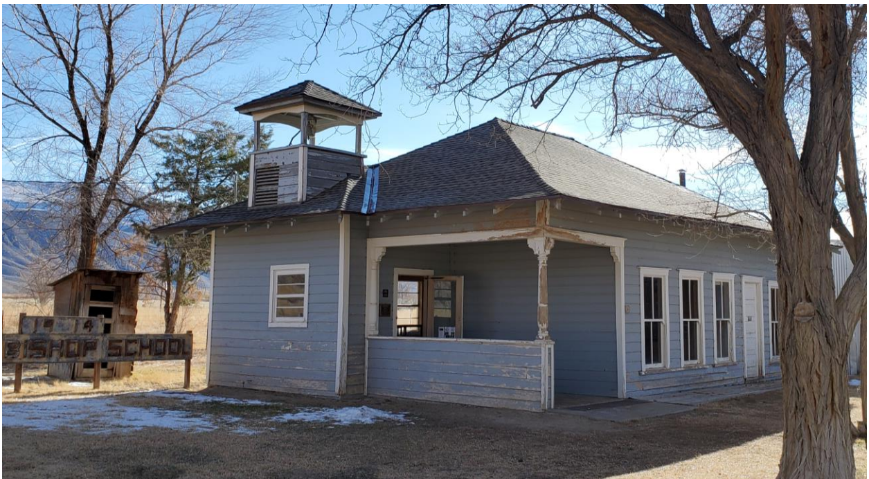
Next up, scraping and paint planned for summer 2022.
