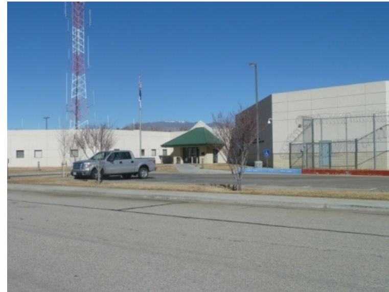
Sheriff Jail ADA Retrofit
