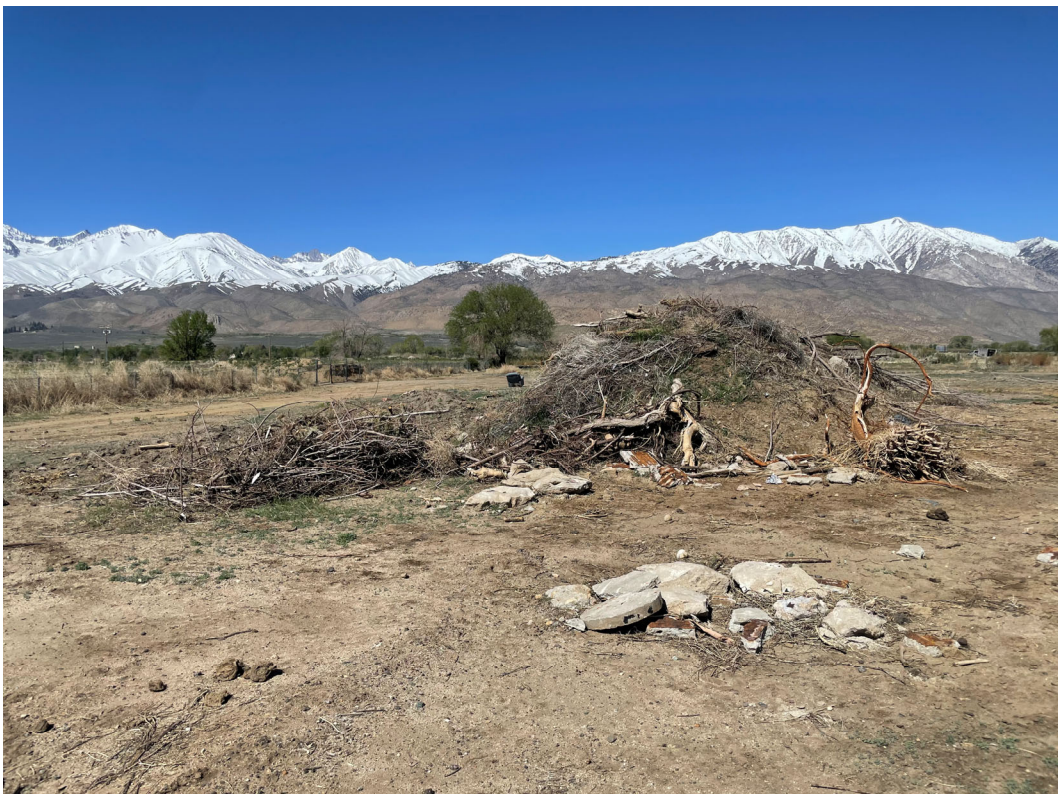
Central location looking west at concrete debris and spoils piles.
