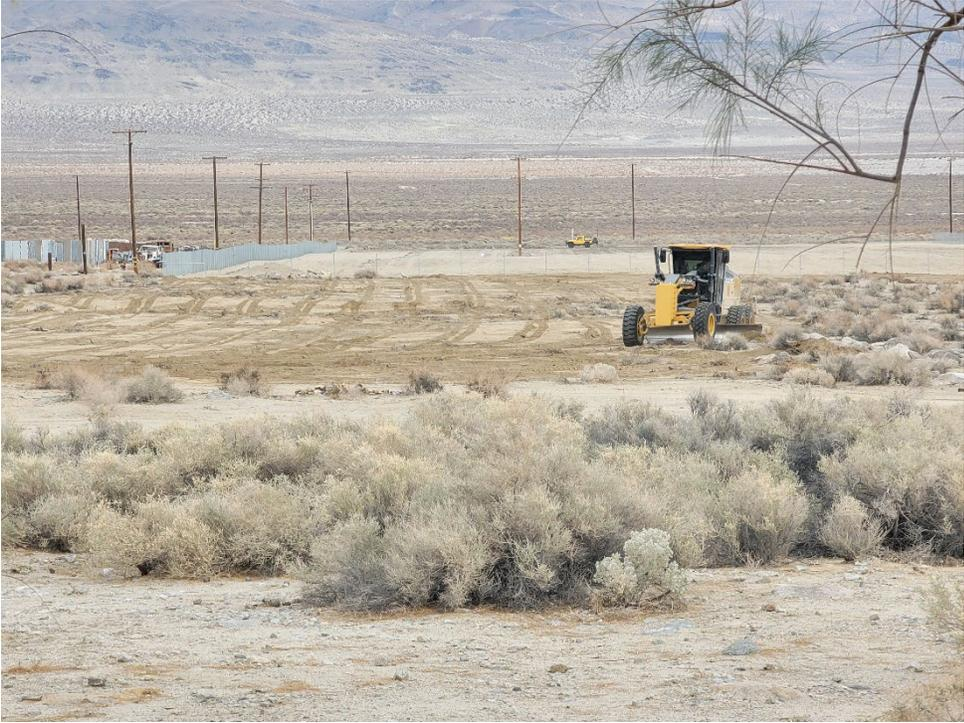
March 19 Photo at Ground Level looking East across Permit area of REP 2022-01 after stripping of land. Note the large depth at which the grading dug into the topsoil.
