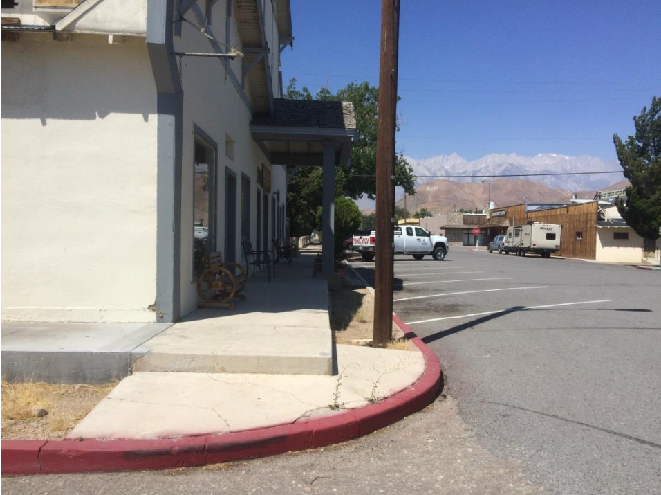
Photo 6: Non-ADA compliant curb
