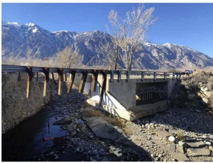
View of existing failed bridge over Pine Creek and abutment to be removed.
