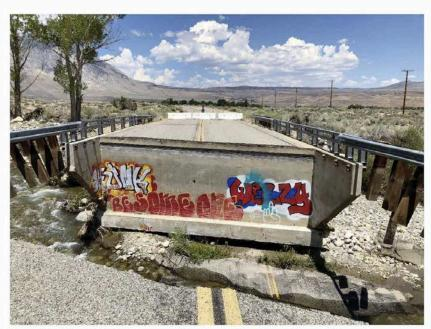
View of existing failed bridge over Pine Creek. A portion of the existing bridge abutment is located within the OHWM of Pine Creek.
