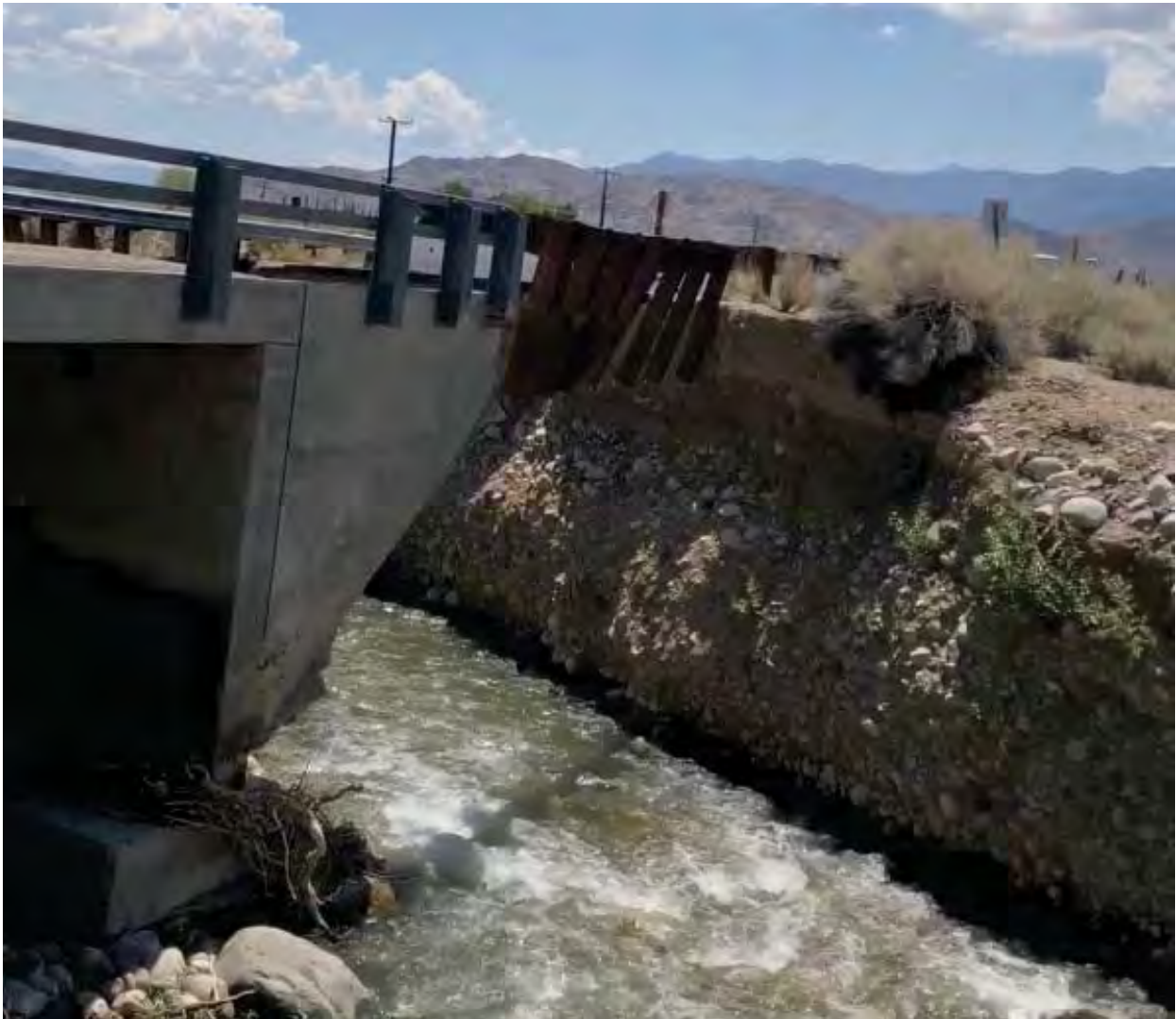
Figure 5 – Failed South Abutment, 2018
