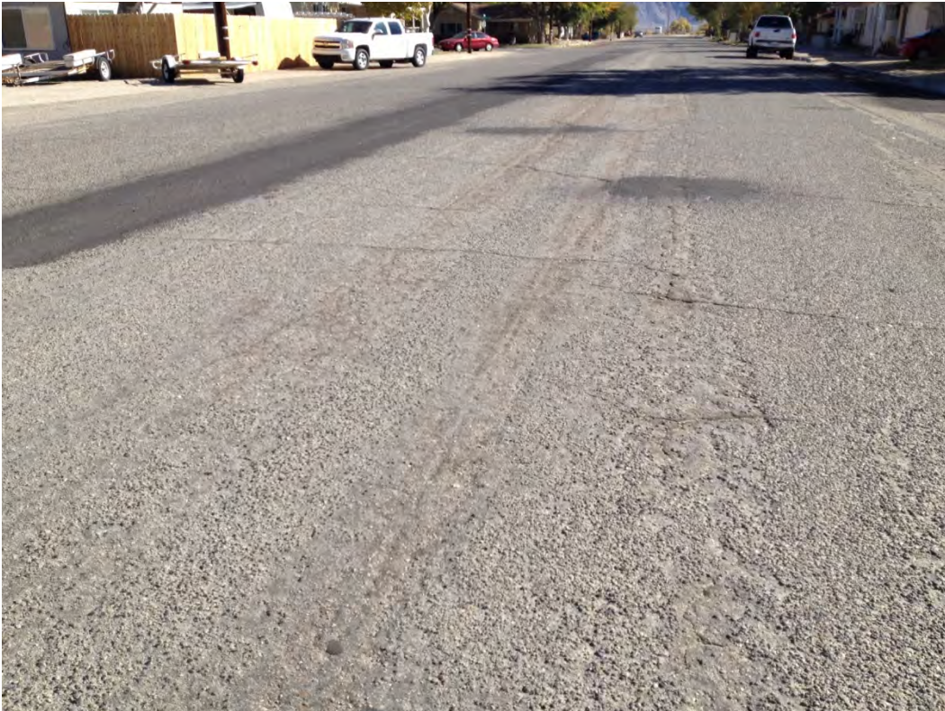
E. Mountain View St.
