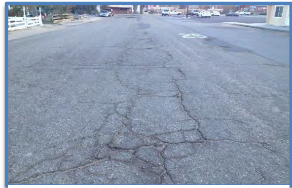
Figure 3 Example of Cracking Pavement, typical
