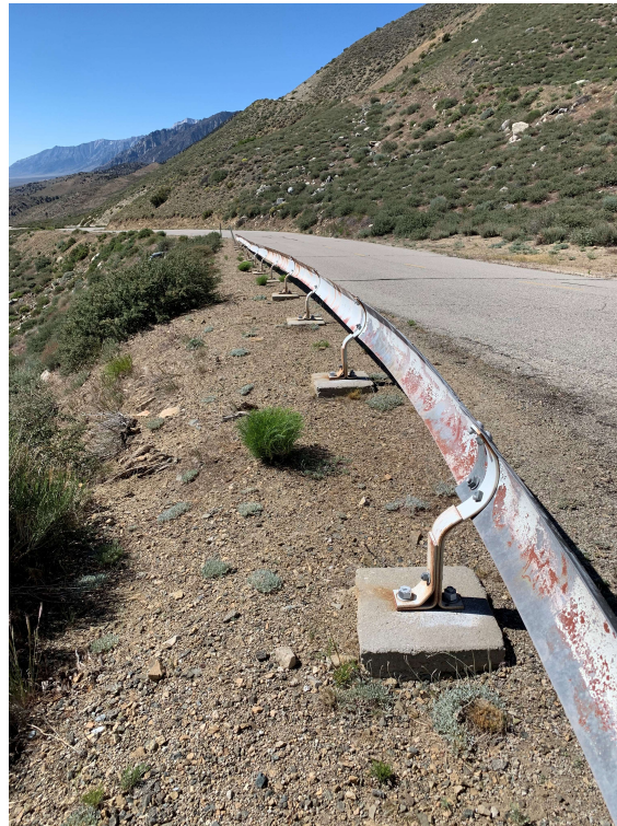
Site 4 - 163 LF of tangent with taper note exposed footings
