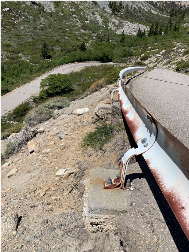
Site 16 - 238 LF Outside Curve
