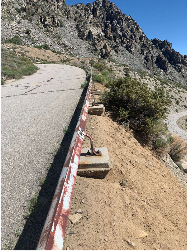
Site 10 - 260 LF Outside Curve
