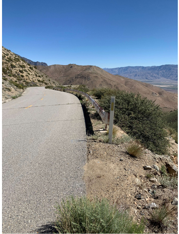
Site 6 - 163 LF Outside Curve
