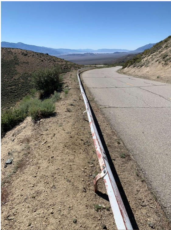
Site 3 - 206 LF Outside Curve
