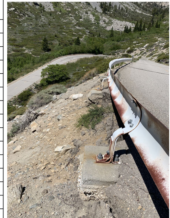
Existing Guardrail at Site 16
