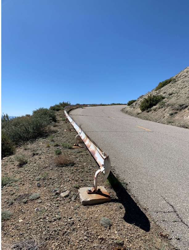
Site 5 - 217 LF of Outside Curve
