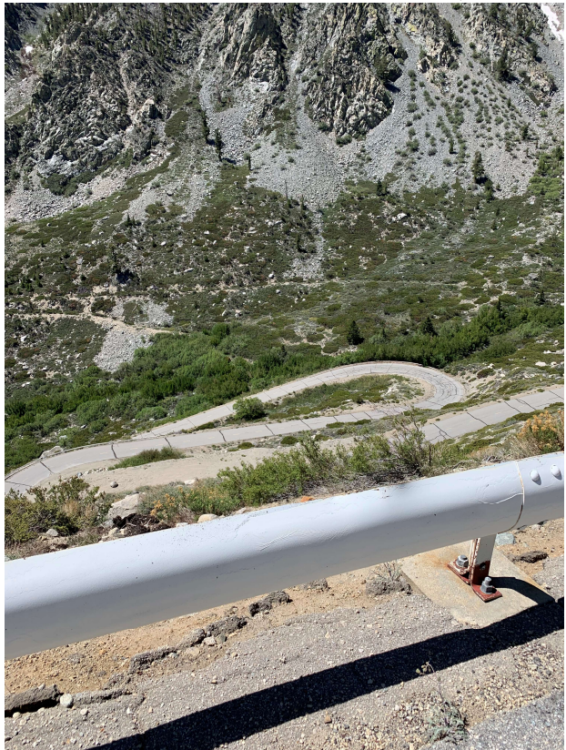
Site 18 - 488 LF Outside Curve
