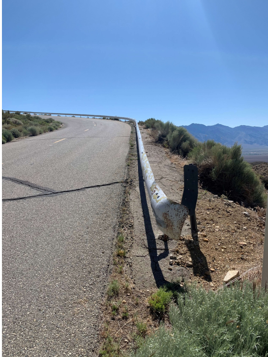
Site 1 - 488 LF Outside Curve
