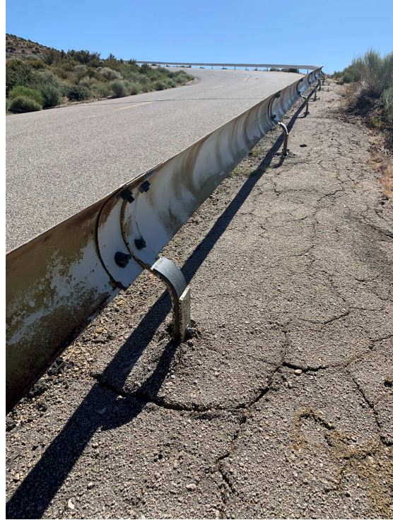
Site 1 - Variable shoulder condition
