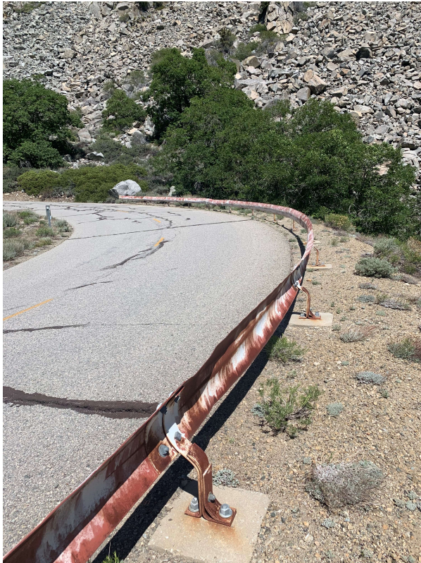
Site 11 - 238 LF of Outside Curve
