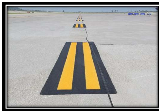
Image 5. Taxiway Edge Marking
