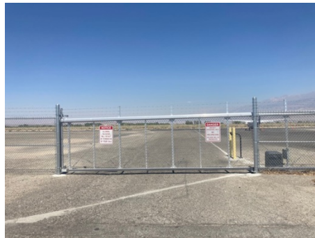
Image 2. Terminal Area Security Gate (Gate No.1)
