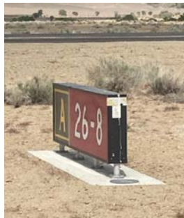
Image 15. Runway Hold Position Sign
