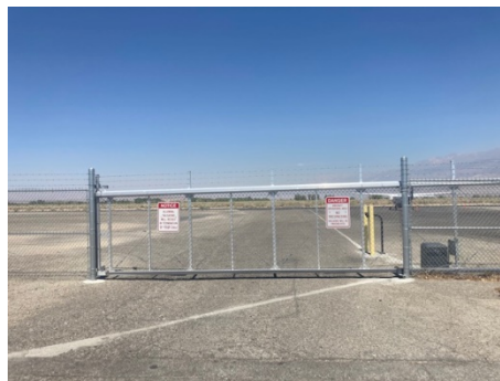
Image 2. Terminal Area Security Gate (Gate No.1)
