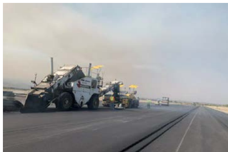
Image 14. Paving operations on Runway 12-30
