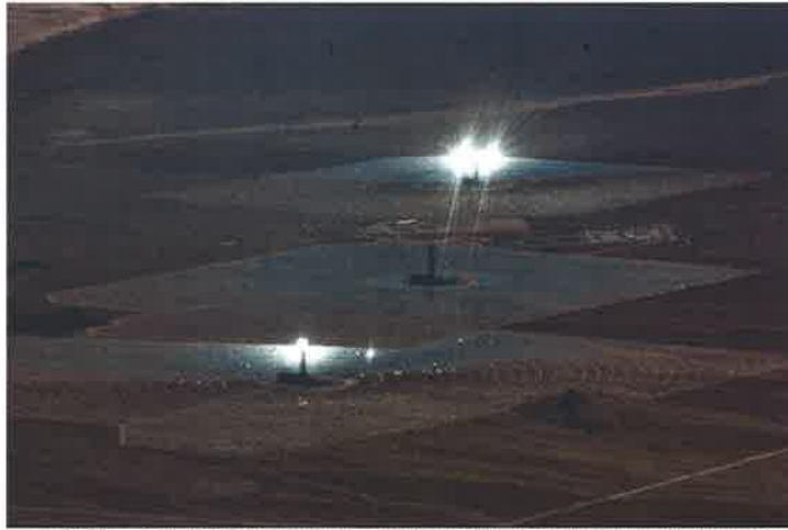
Photo 2. Photo of the ISEGS site taken from the north. From left to right: Tower 3; Tower 2, not in operation; and Tower 1. The photographer's position in relation to heliostat position and orientation results in no DSRH from Tower 3, but strong DSRH from Tower 1 which causes disability glare.
