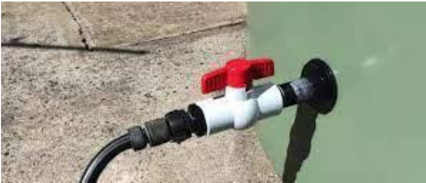
Watertight seal with attached ball valve on the side wall of a tank
