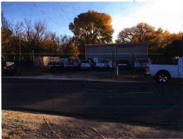
Public Works Building with unpaved lot
