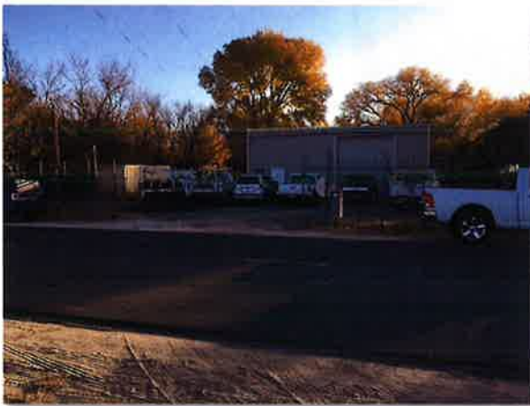
Public Works Building with unpaved lot
