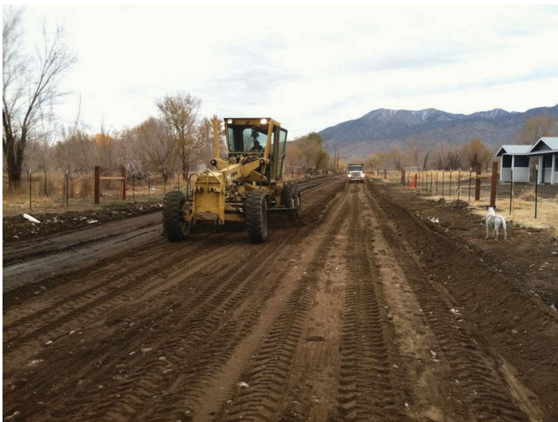
Construction of an interior road on Bishop Reservation in 2013
