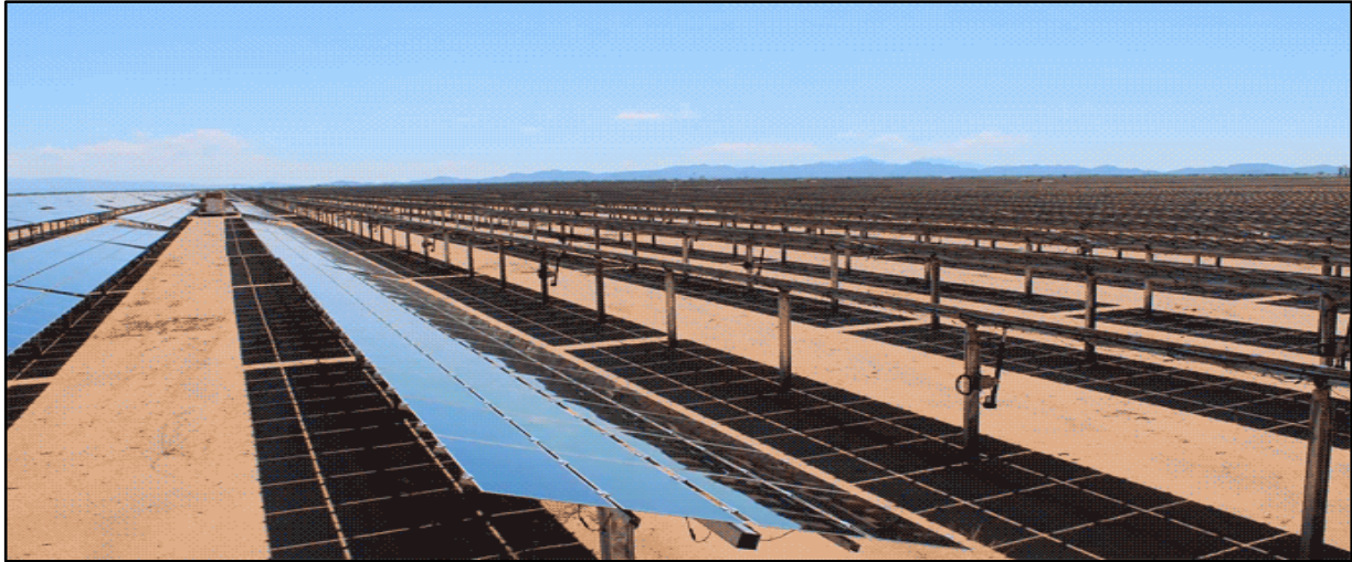
Figure 7-3. PV Module Tracking
