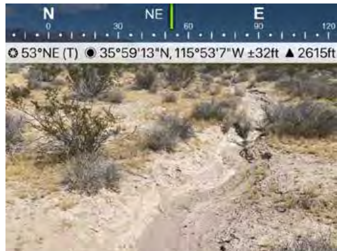
Photo 12. Drainage 217, facing upstream.
