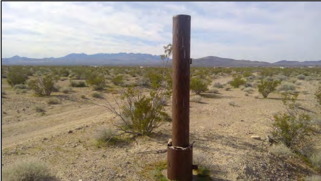
20: Abandoned domestic/ irrigation water supply well located on the intersection South Mcr928200 Road and Avenue D
