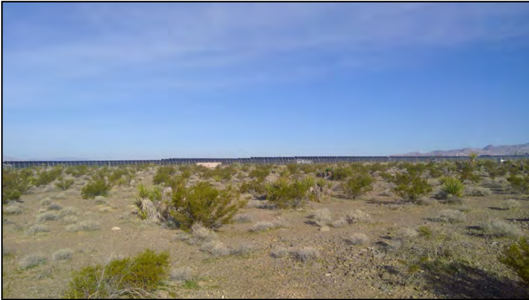
5: View to the north of the Site and Yellow Pine Energy Center (Nevada)
