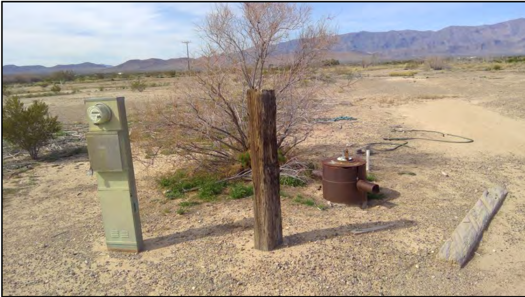
17: Abandoned water supply well and electrical box located on the eastern side of the Site
