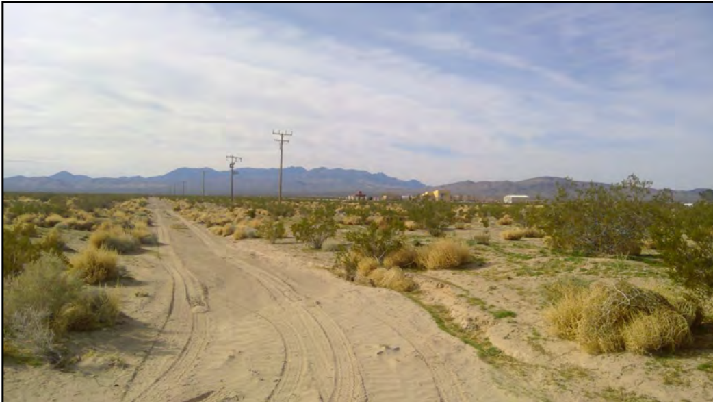
22: Telephone/ electrical lines located on the adjacent property to the south
