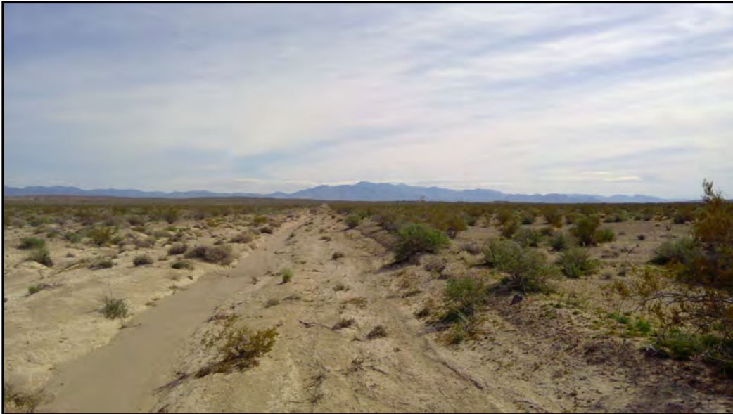
16: Typical condition of the unpaved roads located on Site
