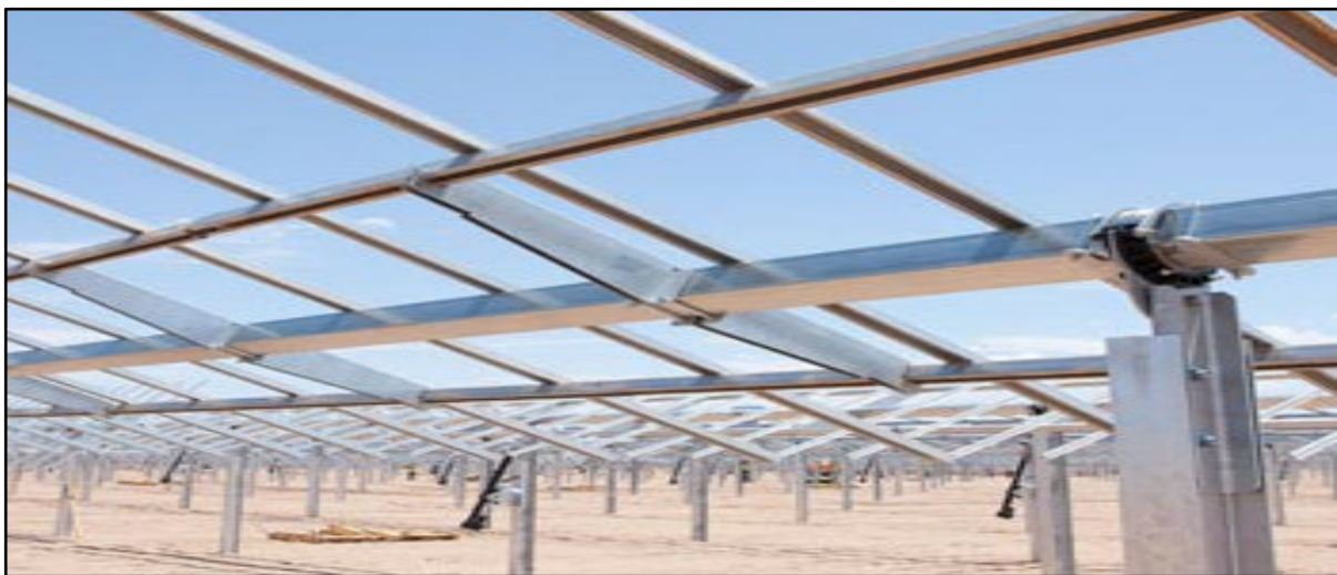
Figure 7-5. Tracking Mounts and Installation
