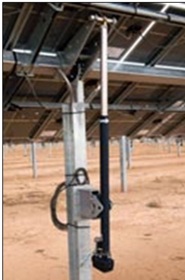
Figure 7-2. Solar Tracker and Actuator
